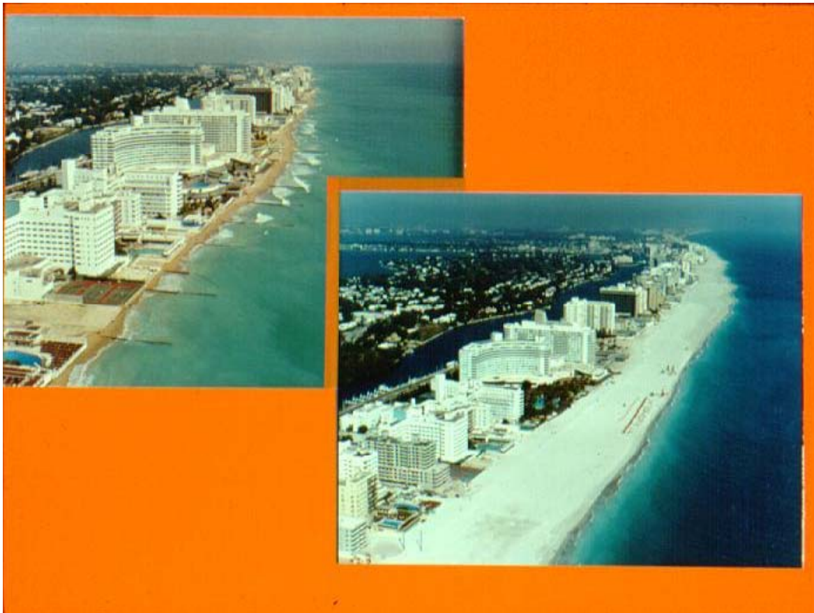
Figure 18-2. Beach renourishment project--Miami Beach, FL (Jacksonville District)
